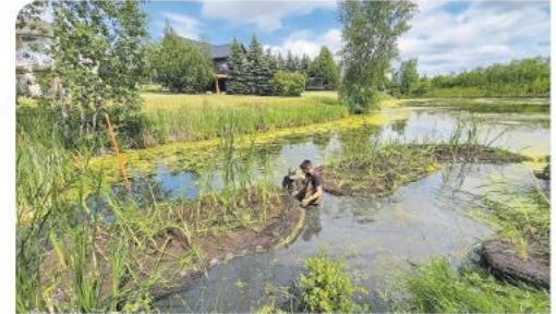
Earlier this month, Richard Grosshans (left) lead researchers from the International Institute for Sustainable Development installing temporary floating wetlands in two retention ponds in East St. Paul. Supplied photo
